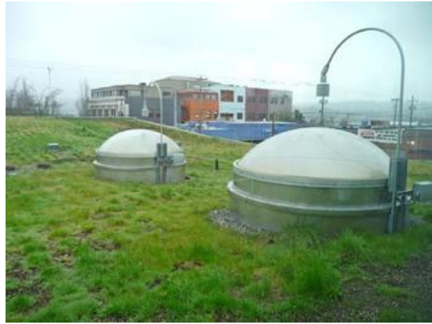
“Green” roof, Ballard branch, Seattle Public Library, with skylights. Image: Christopher Gildow. Used with permission.
