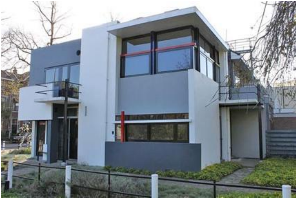
Gerrit Rietveld, Schroder House, 1924. Utrecht, The Netherlands. Image licensed through Creative Commons.
