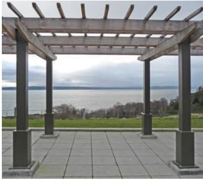
Post and Lintel support in contemporary use. Image by Christopher Gildow. Used with permission.
