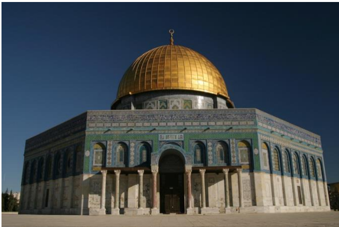
The Dome of the Rock (Qubbat al-Sakhra), Umayyad, stone masonry, wooden roof, decorated with glazed ceramic tile, mosaics, and gilt aluminum and bronze dome, 691-2, with multiple renovations, patron the Caliph Abd al-Malik, Jerusalem (photo: Brian Jeffery Beggerly , CC BY 2.0))
