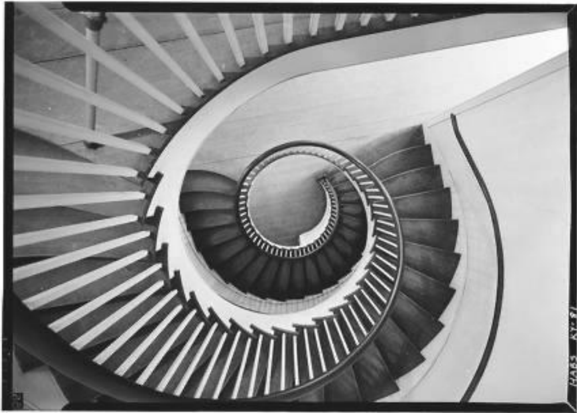
Shaker style staircase, Pleasant Hill, Kentucky. Photo by Jack Boucher, National Parks Service. Image is in the public domain.
